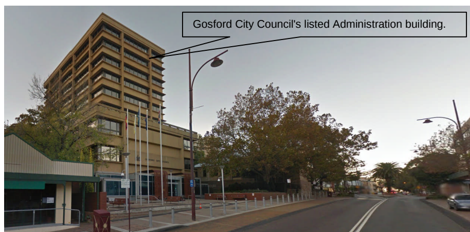
Plate 31: A view looking south on Mann Street toward Georgiana Terrace. (Google Streetview)
