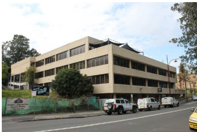
Plate 37: The 4 storey Police Station diagonally opposite the subject site is currently the highest building in the near vicinity. (Source - JBA)
